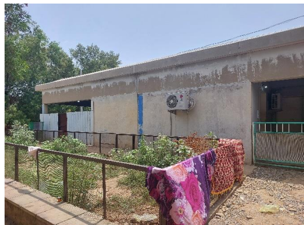
Image 2.7-Pre-cast concrete structure
